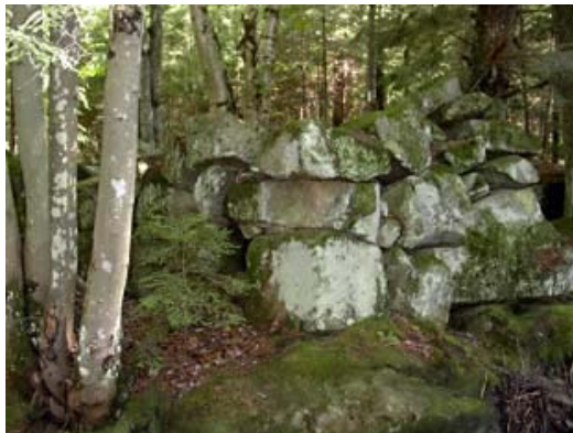
Photo 3: Remnants of the stone retaining wall
