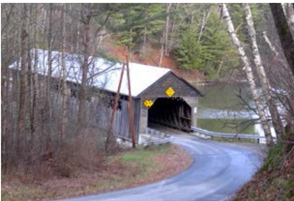
Photo #5, Edgell Covered Bridge
