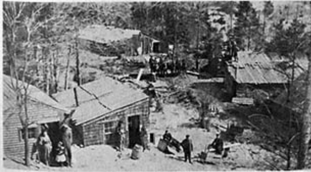
Photo #3 , from Patterns and Pieces p. 35: Piper's lumber camp at Hardscrabble near Trout Pond
